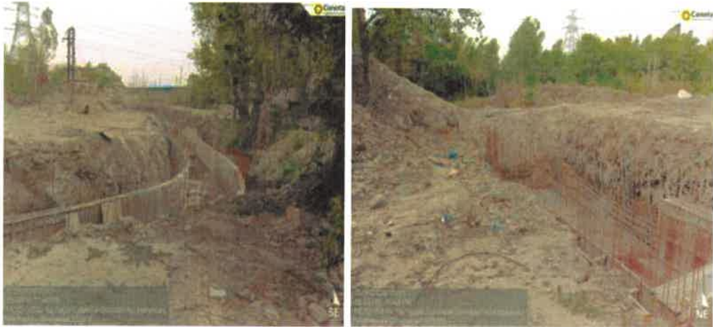
Figure:- Construction of drain.
