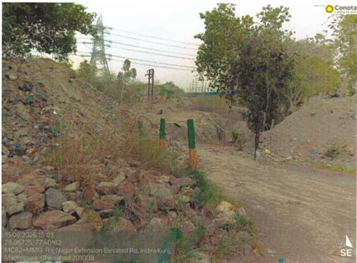
Figure:- Heap of Soil after digging drain
